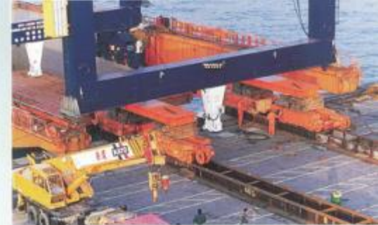
Waterside sill beam ride on ship's deck
