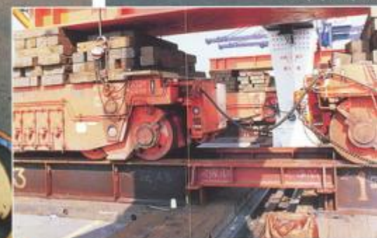
Preparation for lowering onto quay rail system
