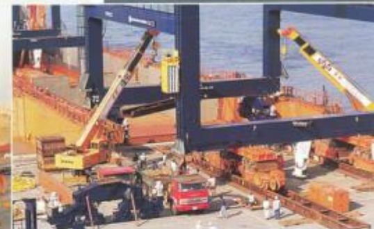
Preparation for lowering onto quay rail system
