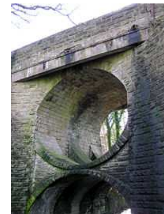
Telford's circular-arch roadbridge in Bannockburn, Scotland
