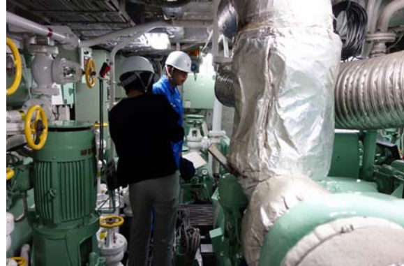
Photo 2. Observation of engine room
